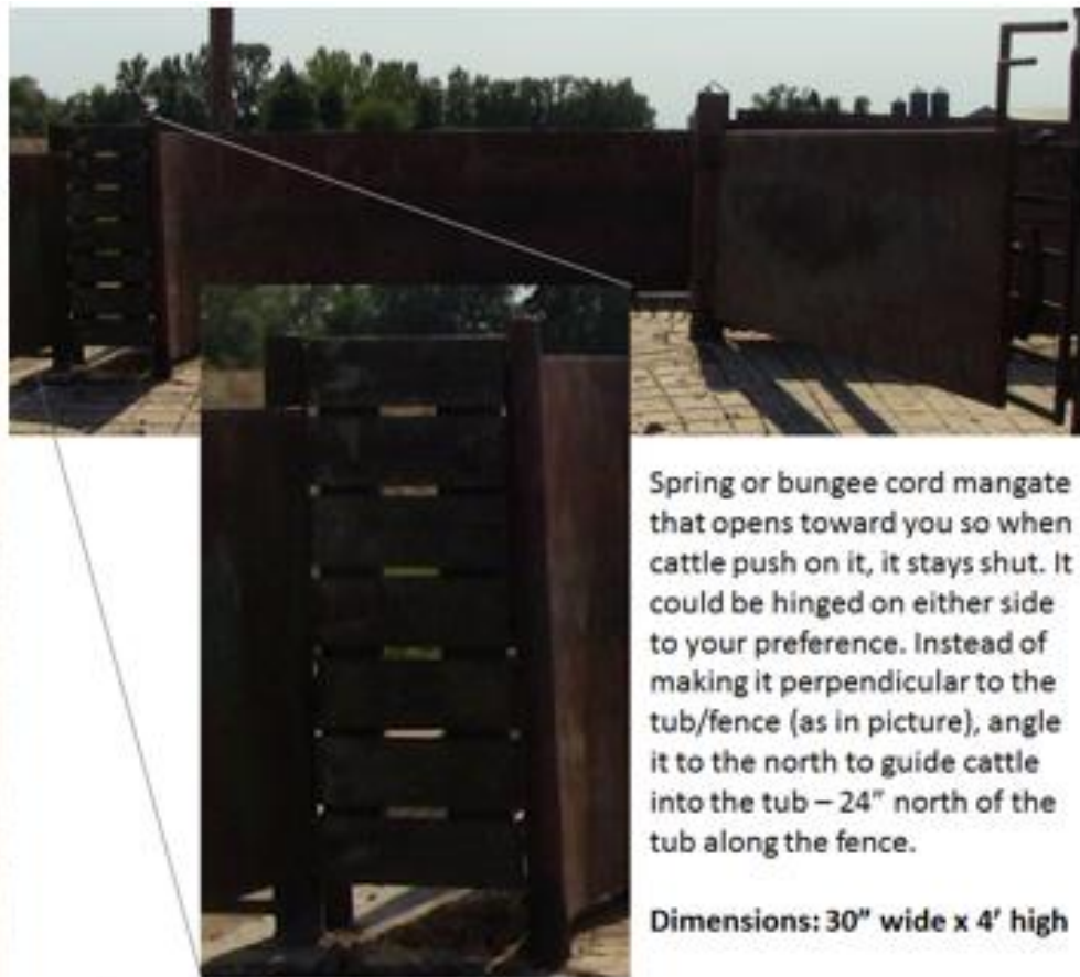
Figure 5: Location and description of the mangate on the east side of the tub.
